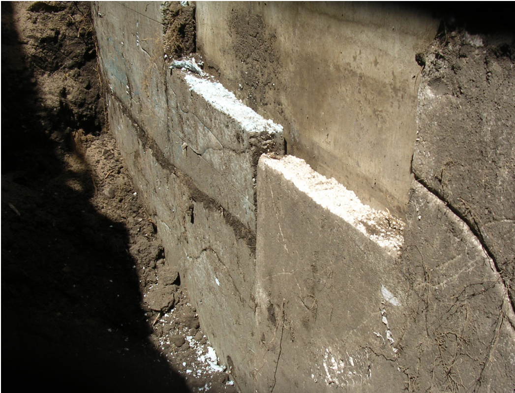
Figure 2. XPS and molded polystyrene below grade insulation
