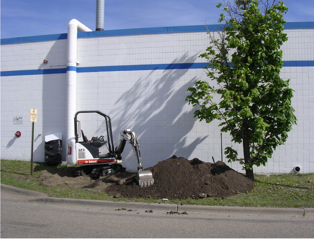
Figure 1. Excavation of insulation samples after 15 years
